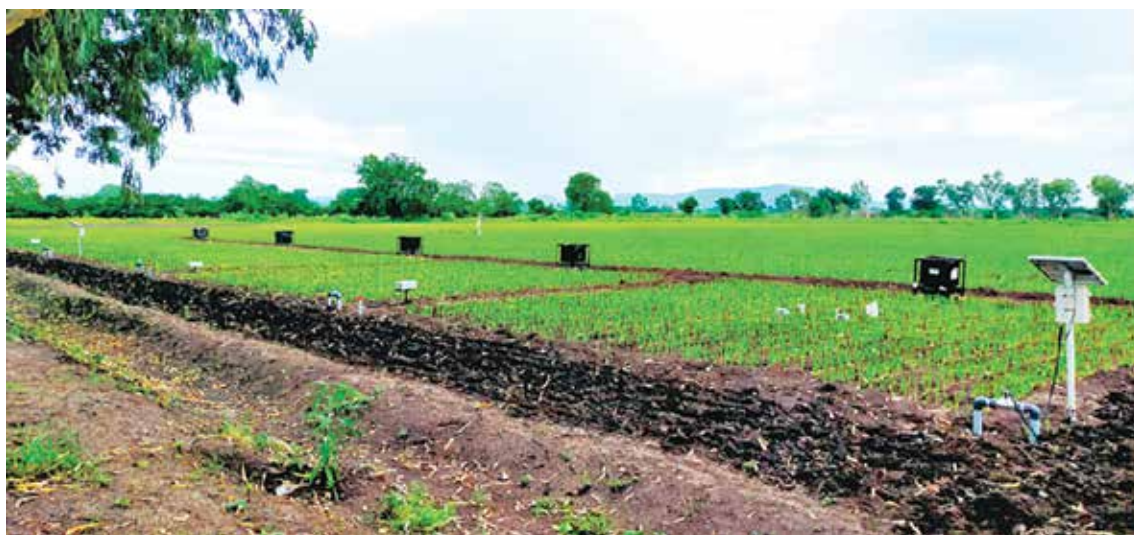
Field Installation of IoT enabled Automatic Pump Controller for Multiple plots (SmartPIS system)
